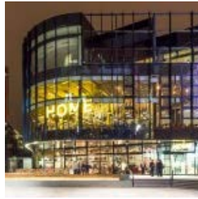
MECANOO COMPLETES HOME CULTURAL CENTER IN MANCHESTER
